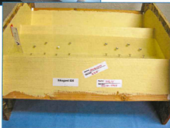
Photo 21 – Fastener sealability testing of liquid-applied flashing mock-ups in progress.
