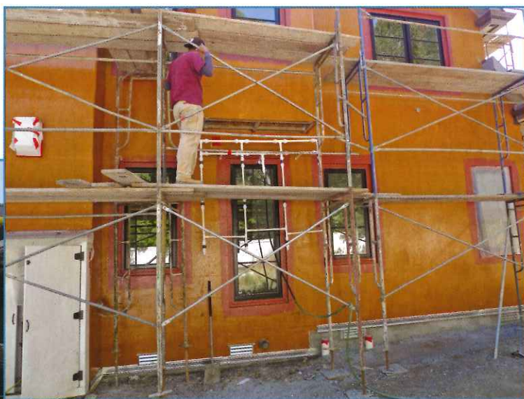
Photo 2 – Fluid-applied WRB, air barrier, and flashings applied to residential project.
