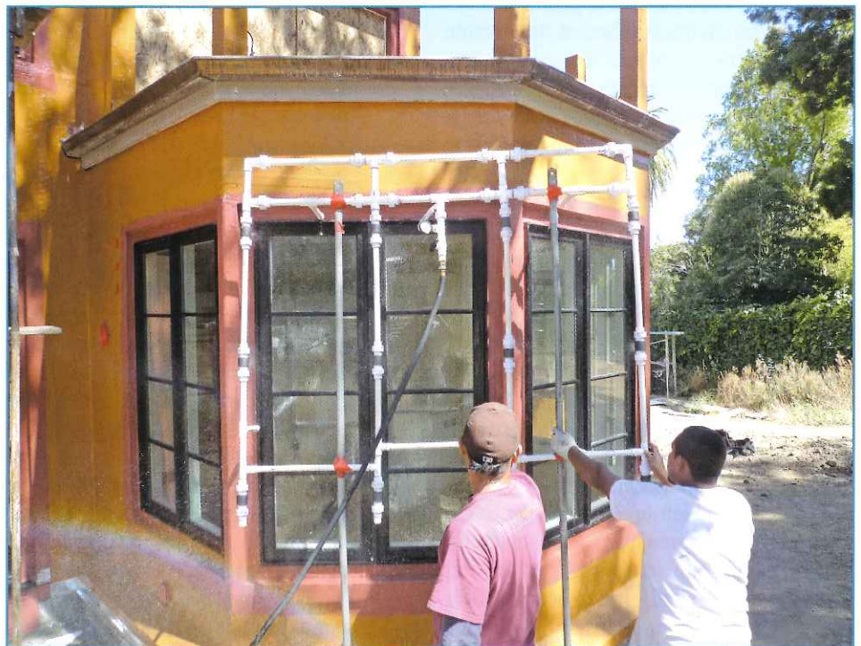
Photo 23 – On-site water testing of fluid-applied WRB and flashings.
