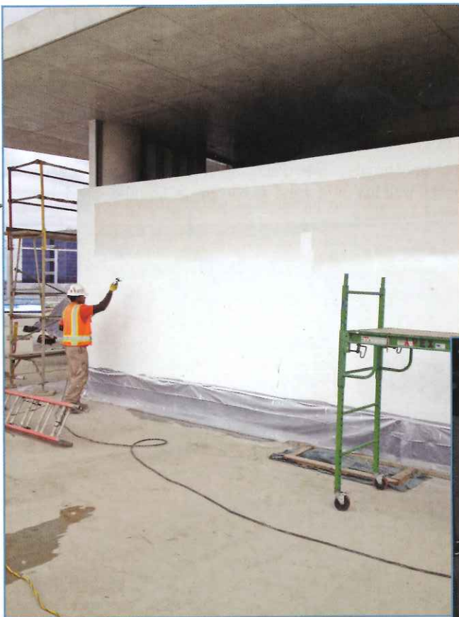
Photo 4 – Fluid-applied WRB being sprayed. Photo courtesy of Dow Corning.
