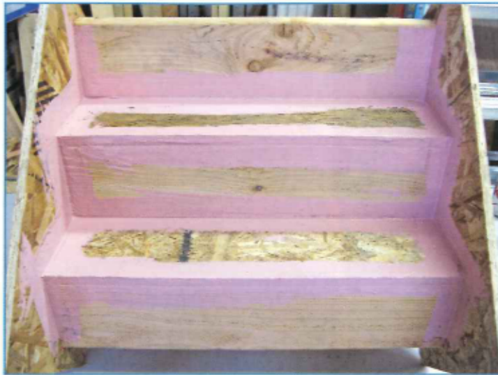
Photo 14 – STP application, best practice. Step 1: Seal joints and seams. Use putty knife to create screed.
