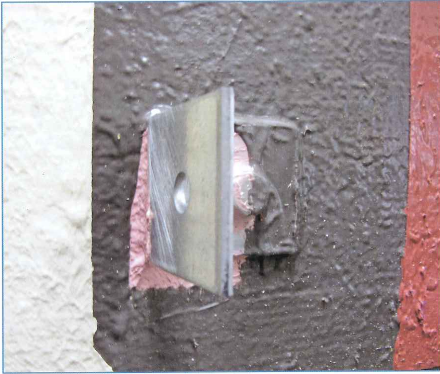
Photo 3 – Fluid-applied WRB and flashings applied to an irregular penetration.
