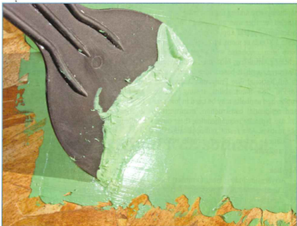
Photo 7 - Silyl-terminated polymer (STP) flashing being troweled.
