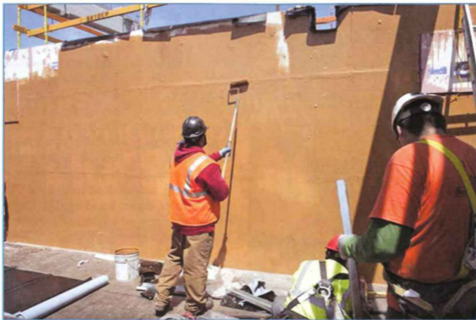
Photo 6 – Fluid-applied WRB being rolled. Photo courtesy of Prosoco.
