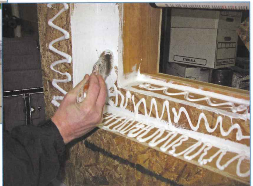
Photo 5 – Fluid-applied WRBs and flashings may be brushed.
