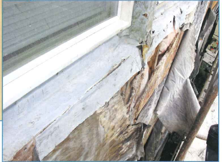
Photos 9 and 10 – The problem child: the typical recessed window. Water intrusion damage from improperly applied or sealed SAF in a typical recessed window flashing installation.
