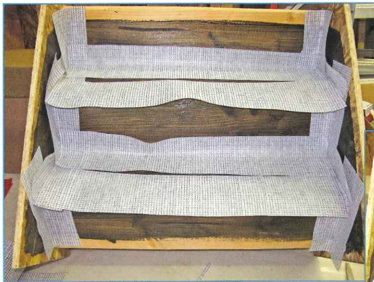
Photo 16 – Some acrylics require fabric reinforcing. Pre-cut fabric is shown.
