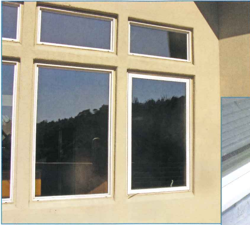
Photos 9 and 10 – The problem child: the typical recessed window. Water intrusion damage from improperly applied or sealed SAF in a typical recessed window flashing installation.
