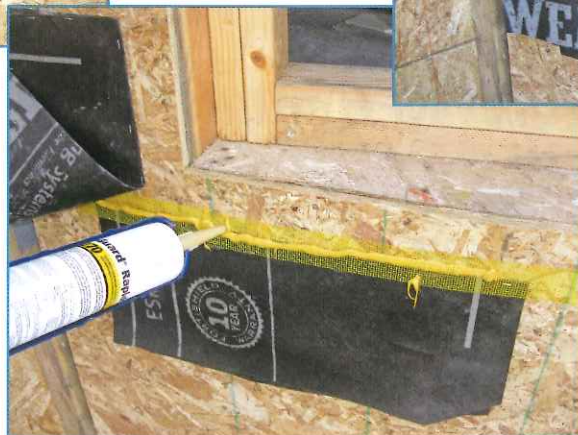
Photo 12 – Recessed window flashing. Step 2: Apply liquid flashing to fabric tie-in transition.
