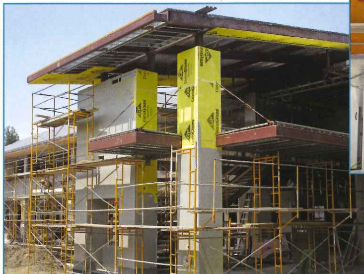
Photo 1 – Fluid-applied WRB and air barrier applied to commercial project.
